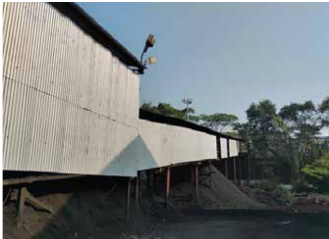
Figure 9: Site Porous walls around the conveyor and stockpile.
